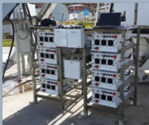
Redundant system controllers for Outdoor PowerMAX
