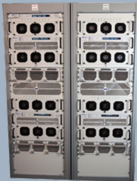
A pair of phase-combined PowerMAX rack assemblies.
